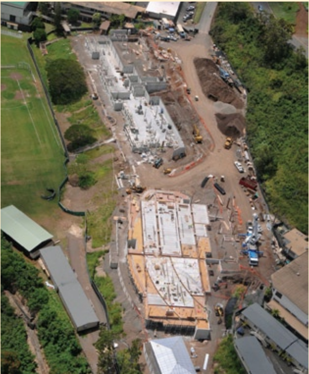
Construction continues on the KS Kapālama Middle School. This photo was taken in April.
