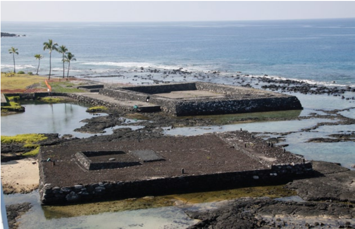
Thanks to the efforts of Kamehameha Schools and the remarkable Hawaiian stone mason Billy Fields and his crew, Hāpaiali'i and Ke'ekū heiau rise once again in this view from the Keauhou Beach Resort in Kona.
