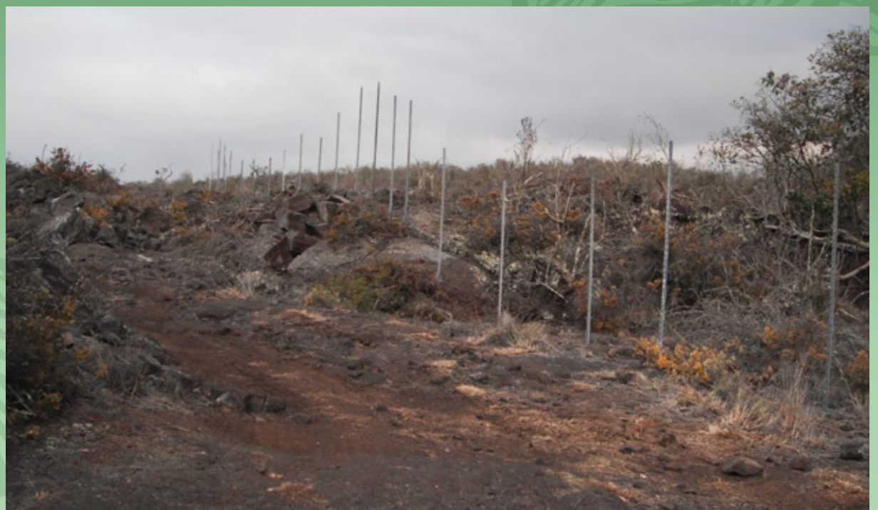
Construction along this fence line will protect the tropical dryland forest from the threat of hooved animals.
